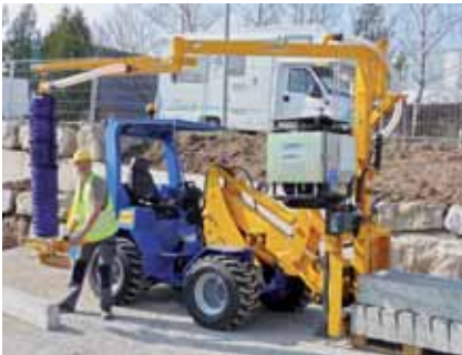
... vacuum laying attachment: safe, quick and efficient – Kerb Stone Installation Machine Jumbo BV-vario.
