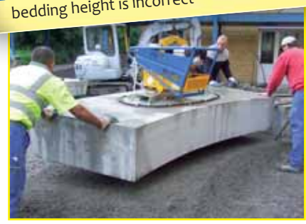
SH 2500 uni b , traditional, strong-as-an-ox unit; part of our product line for 20 years; load classification up to 2,500 kg; powered by a petrol engine
