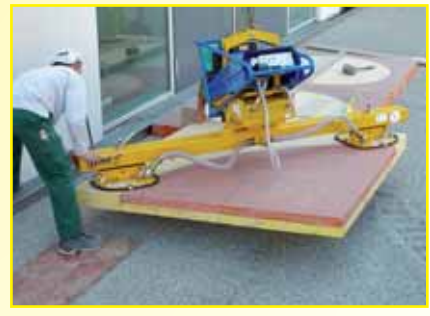
SH 2500 uni b, with Traverse TRA 3000 For installing multicoloured special panels (ca. 2 x 2 m)
