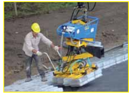
SH 2500 uni b with a special multipurpose vacuum panel. This unit allows 12 embankment pavers with vertical interlock to be taken off a pallet, shifted into running bond and installed after being adjusted to the slope.
