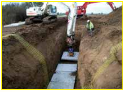
SH 2500 uni b , the greatest amount of freedom for the shovel excavator operator. With radio remote control and a hydraulic control knob. This permits elements to be safely installed even inside hazard areas without additional help.
