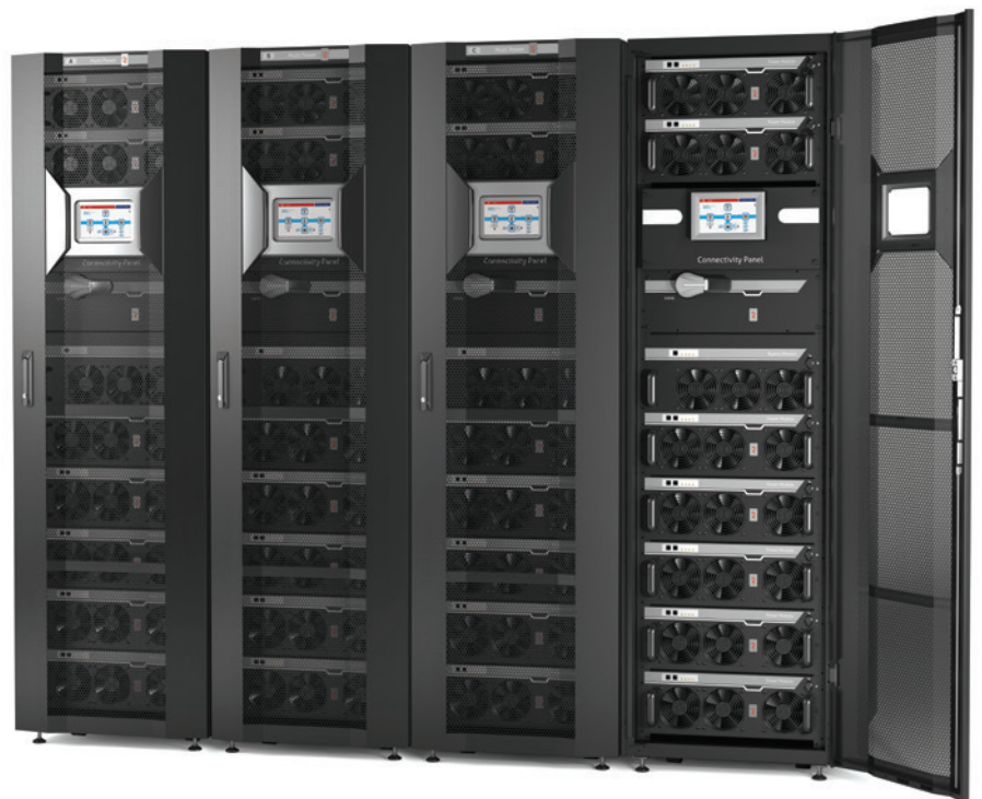
Power Cabinet (1+7 x Power Modules) x 4
